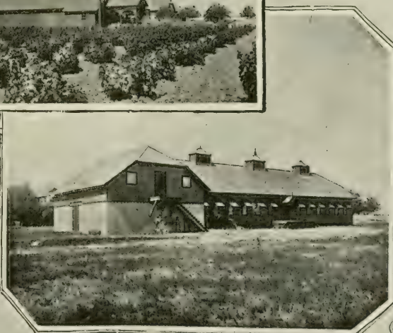
Views from Col. Wm. Forsyth's Raisin Vineyard, Near Fresno: Residence, Lake, Raisin Dryer, Packing House.
